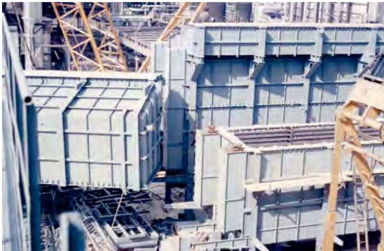
ENICHEM ANIC, Gela (Italy) Delayed Coking Furnace with APH.
