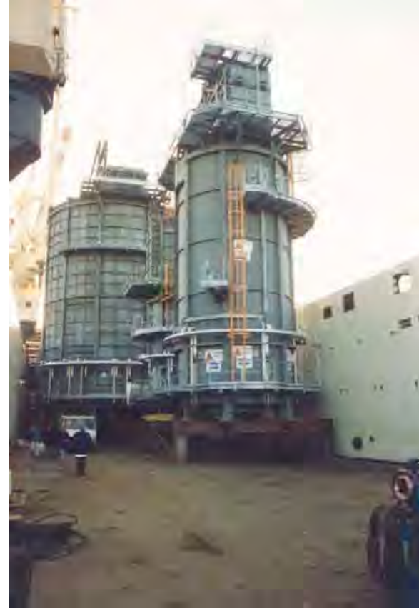
STATOIL, Kalundborg (Denmark) Hydrofiner & Hot Oil Heaters.
